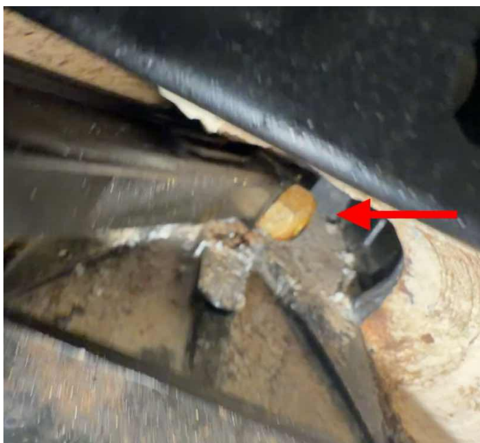
L29. Corrosion to transom assembly steering pin
