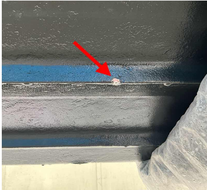
L23. Gelcoat gouge to port side strake beneath waterline
